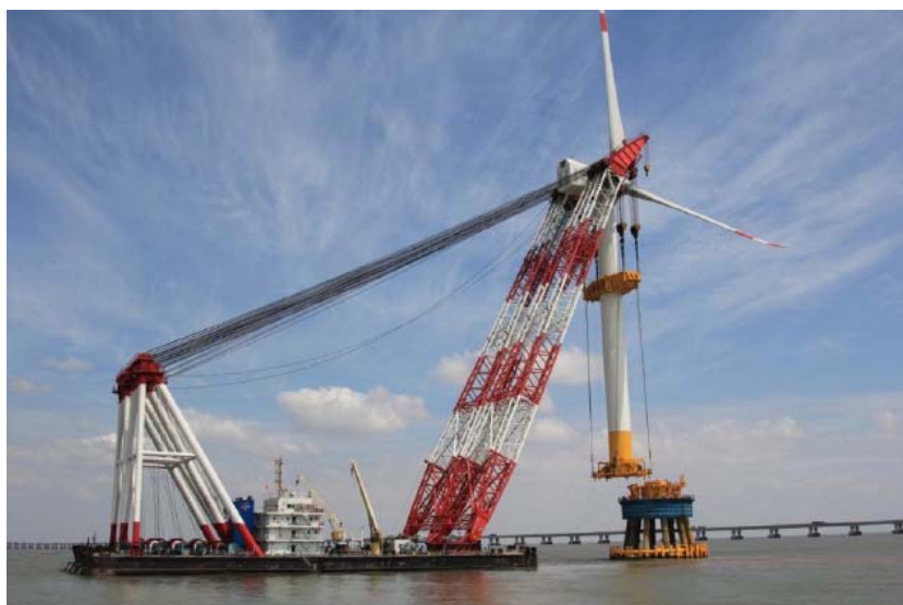
Fig.6.3.2. Installation of Sinovel 3 MW turbine at Donghai Bridge.
