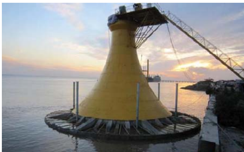
Fig.6.2.12. DaoDa suction bucket foundation, installed in Jiangsu intertidal zone.
