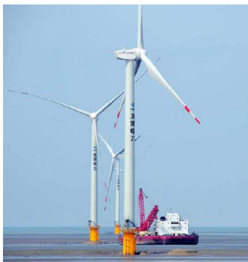
Fig.6.2.6. Monopile foundations installed in the 150MW Longyuan Rudong intertidal project
