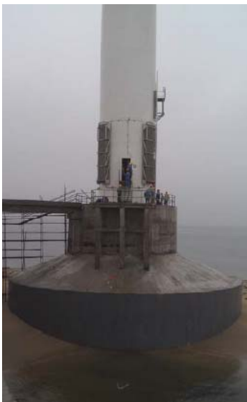
Fig.6.2.9. Fuqing 5 MW prototype foundation (intertidal)
