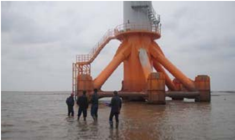
Fig.6.2.7. Multi-pile foundation installed in the Longyuan Rudong 150MW intertidal project.
