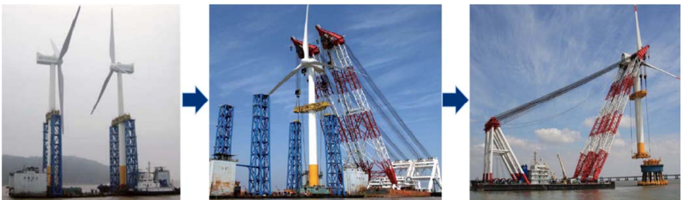
Fig.6.3.5. Installation of Sinovel 3 MW turbine using ZPMC vessel at Donghai Bridge
