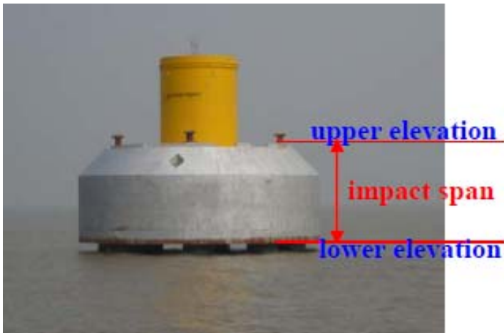
Fig.6.2.5. High-rise pile cap
