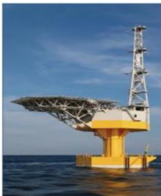
Figure 17. Offshore substation equipment (Fukushima demonstration project) 56
