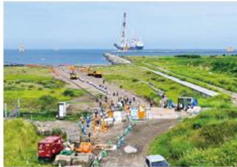
Submarine Cable Laying Work
