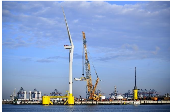
Figure 20: Kincardine 9.5MW turbine installation (Principle Power)
